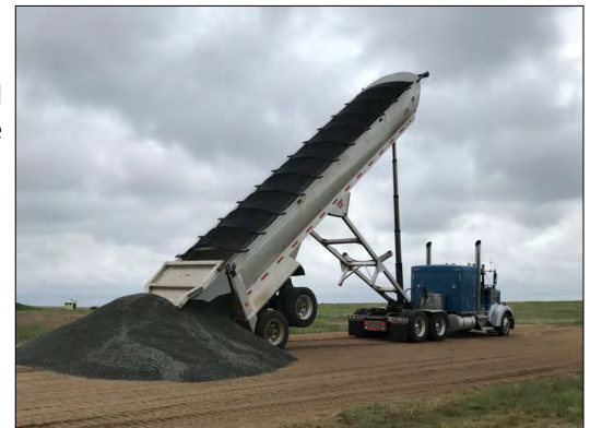
Delivery of 54 ton of 3/8" chip rock for the 500-yd and 600-yd firing lines on the High Power Range.
